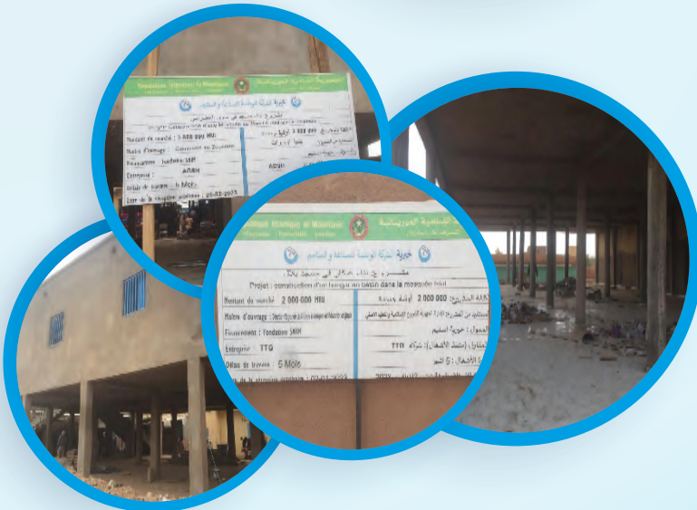
Construction of a mosque in the Hadrami market and the extension of Bilal mosque in Zouerate.
